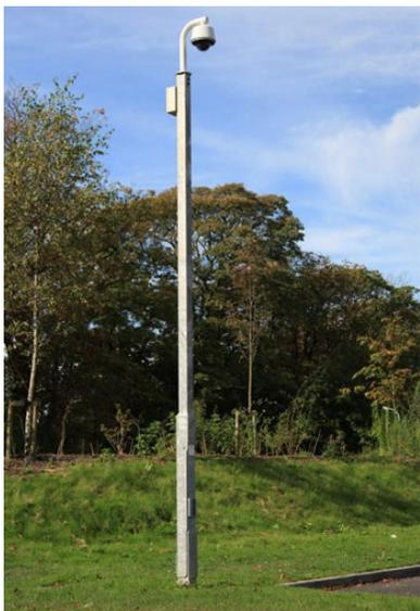
Outdoor IP camera installation is completed in one of two ways, either mounted on a pole or on the side of a building. A large facility can have dozens of cameras mounted in various locations using a variety of methods. We will be focusing on the pole type mounting for the outdoor cameras, as they are the most acceptable to damage from a surge.
