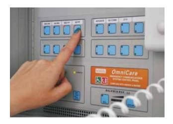
The Omnicare system was the first of its kind when introduced in 2007 as a combined EVC system. Since then it has been installed worldwide and has become the system of choice for many. The system now includes a three-part toilet alarm kit which, like all of the remote units, is powered from the line.
