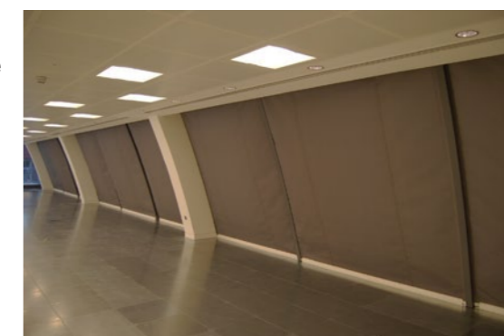
Removable, reinforced suspended ceiling with stall plate
