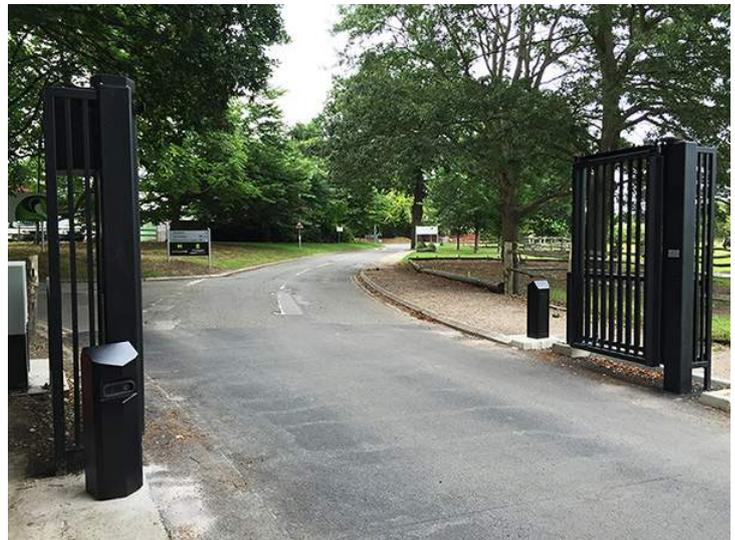
Two RoadWolf ANPR Bollards were installed to log the details of any vehicles attempting to gain entry or exit the site out of hours.
